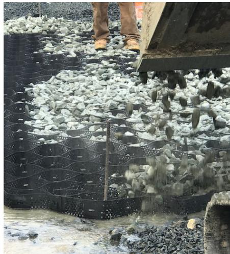
Visible ponding that Geoweb will protect against after installation
