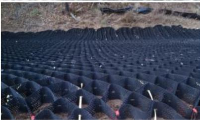
GEOWEB® system with tendons every 3-cells expanded down the slope.
