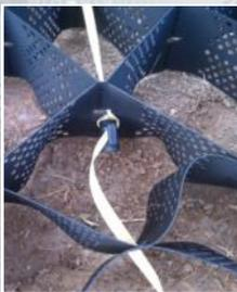
Left photo : A tendon and ATRA® load transfer clip are passed through the GEOWEB® cells.
